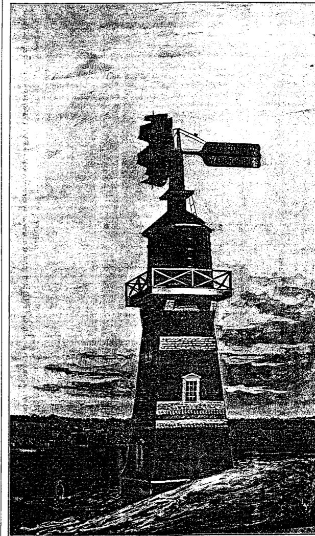
"Fairview" Water Works.
